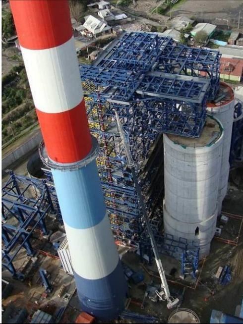
**DESIGN FOR GYPSUM SILOS IN REINFORCED CONCRETE AND METAL BUILDING FGD IN HIGH-RISK SEISMIC TERRITORY**
